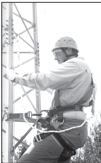
Photo 4: Our climber on the tower. His positioning lanyard is attached to the tower and the fall arrest lanyard is hooked to the tower above him.
